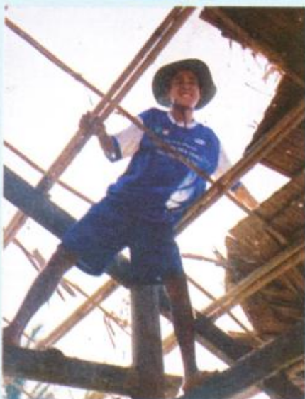
Building a house for poor people
